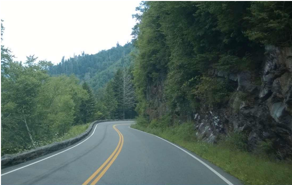
Figure 25. Horizontal curve with limited sight distance
